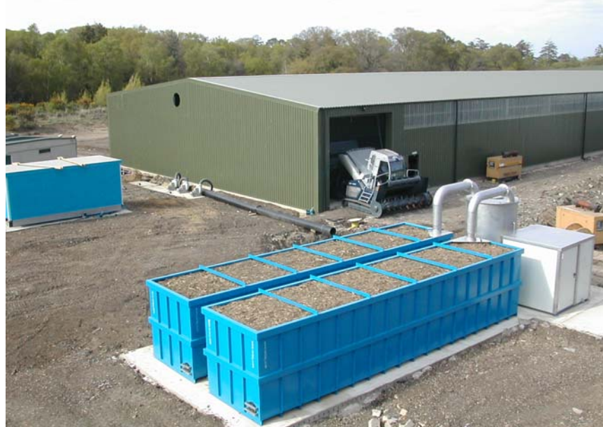
Plate 1 New Earth Technology showing biofilter and scrubber in foreground and composting hall in the background with the windrow turner emerging from the hall.
