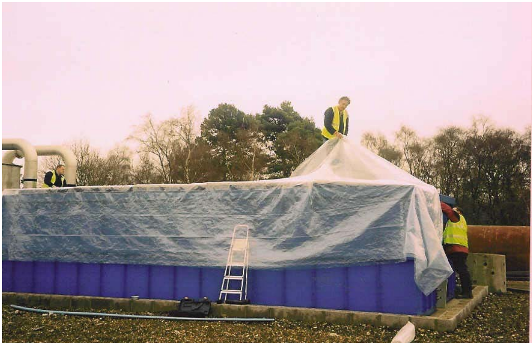
Plate 4. Preparation for capturing gaseous emissions from the biofilter
